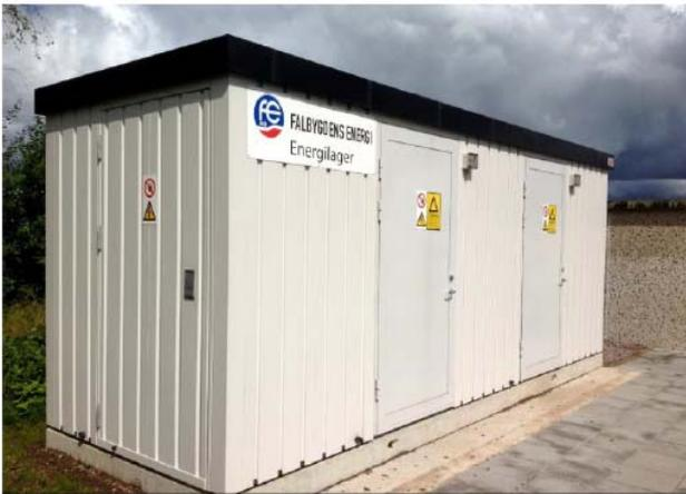
**Figure 3 - The 75-kW battery storage in Falköping – Paper 0586**
