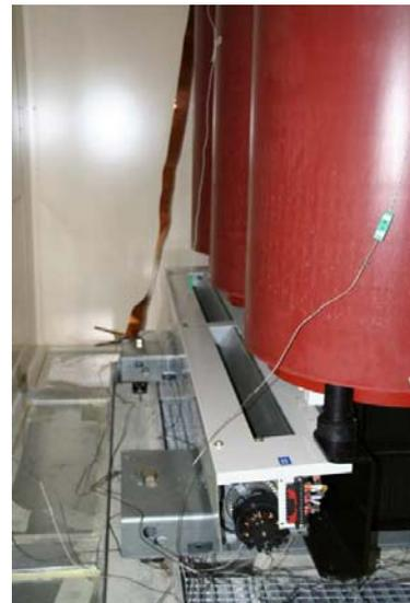
**Fig. 29:** from paper 0625 – Radial ventilation system at the bottom of a dry-type transformer
