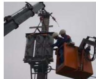
**Fig. 35:** from paper 0521 – Installation of a pole-mounted dry-type distribution transformer
