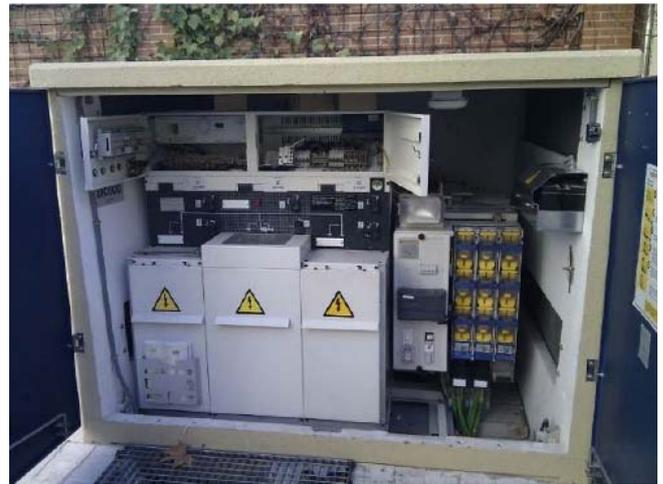
**Fig. 22:** from paper 0519 – Overview of a smart secondary substation
