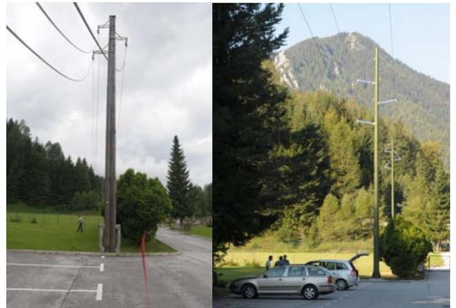
**Fig. 15:** from paper 0294 – Line before and after upgrading from 35 kV to 110 kV
