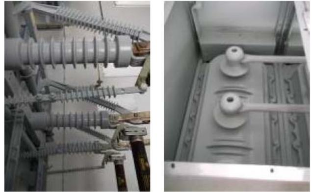
**Fig. 14:** from paper 0694 – RTV silicone application on insulating surfaces
