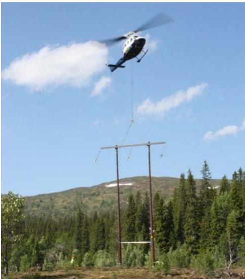
**Fig. 11:** from paper 1393 – Helicopter used for transport and placing of pre-assembled poles
