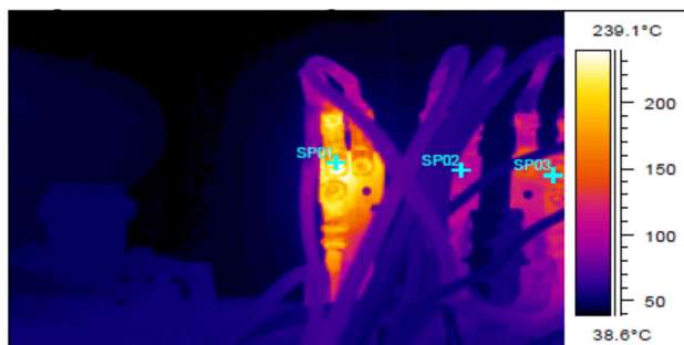
Fig. 3: Transformer bushing, increasing temperature in all three phases
