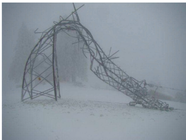
Fig. 10: Ice caused damage on an overhead line
