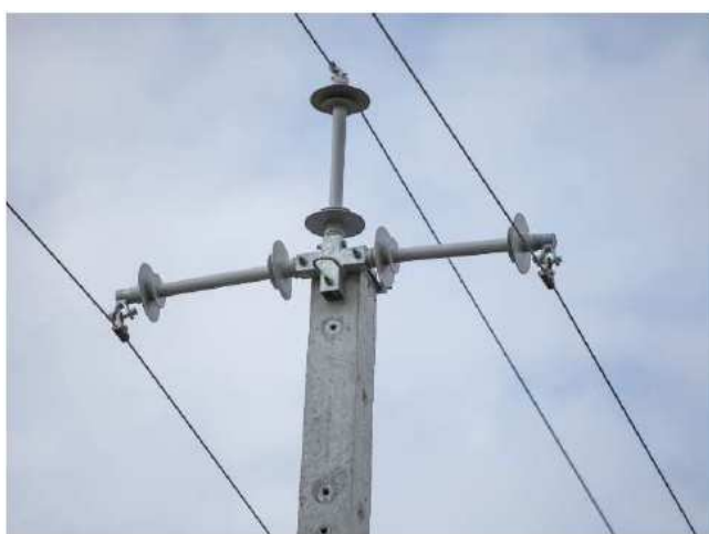
Figure 11 from Paper 1288: Bird-friendly support structure with insulated cross arms
