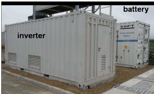
Figure 1 from paper 0775: Picture of the battery and the inverter at the EDF concept grid platform
