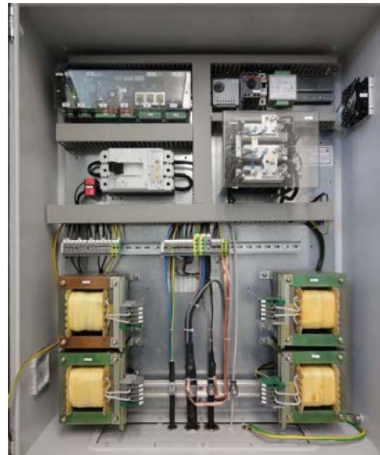
Fig. 11: Realized thyristor-controlled HPCI
