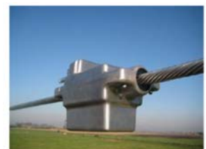
Fig. 3: Installation of smart grid sensor Ampacimon on a 150kV line
