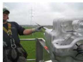
Fig. 3: Installation of smart grid sensor Ampacimon on a 150kV line
